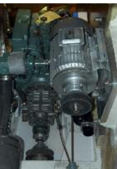
Diesel electric and hybrid installation.
